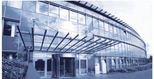
Basler AG Germany, Headquarters
