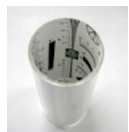
sample of pipe inspection
